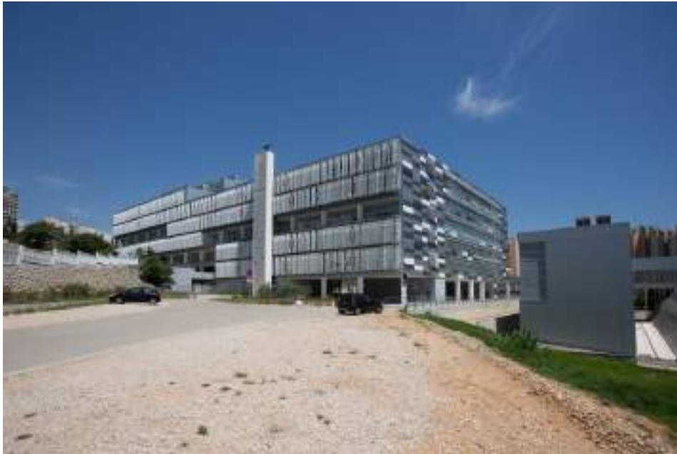
South West side of Faculty building, University of Split Faculty of Chemistry and Technology, Split, Croatia
