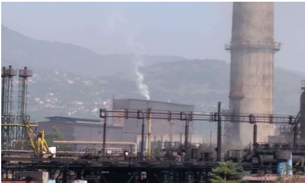
Figure 2. Western layout view from a broken portal crane
