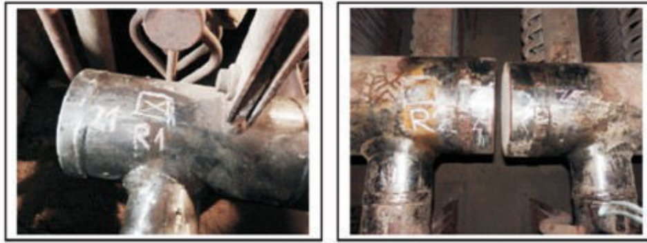
Figure 1. Place of taking the replica at the header of KP 13
