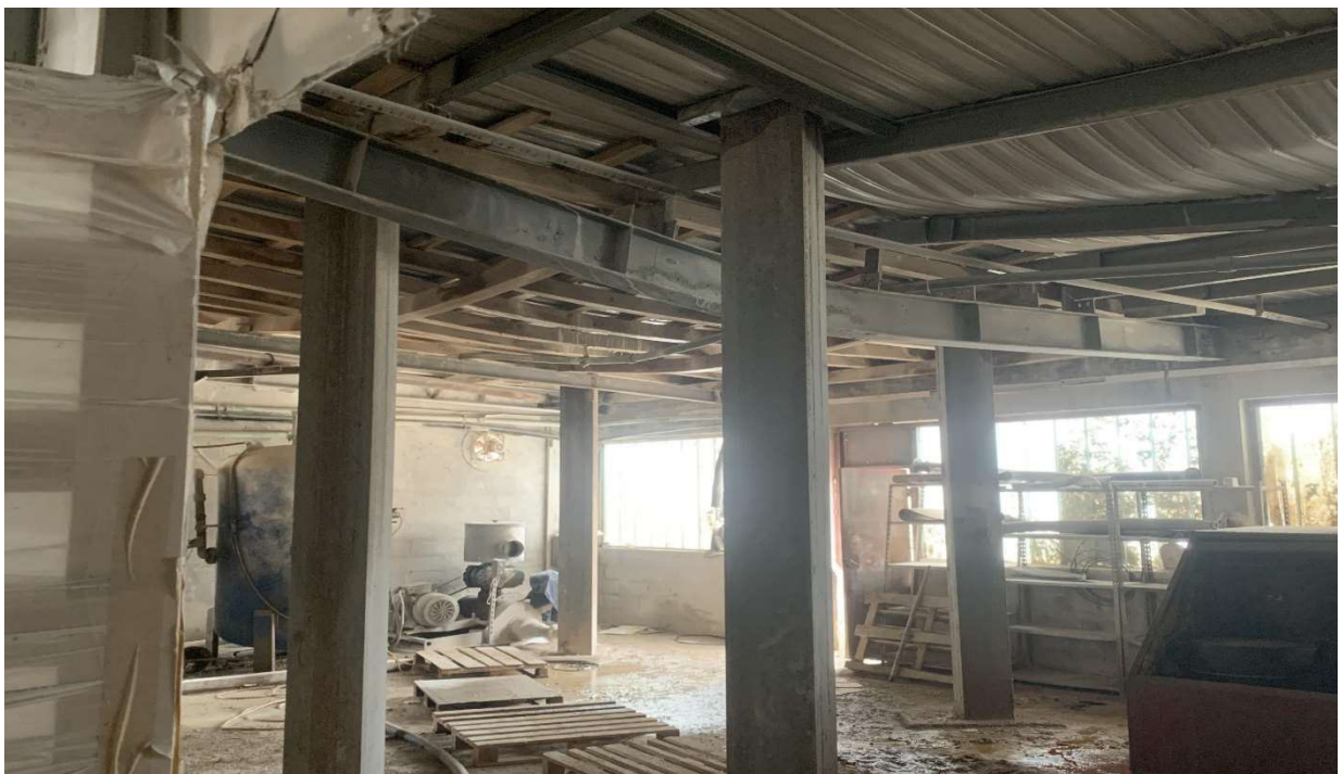
Figure 10. Detailed position of the wooden section supports to plastically deformed sections & roof
