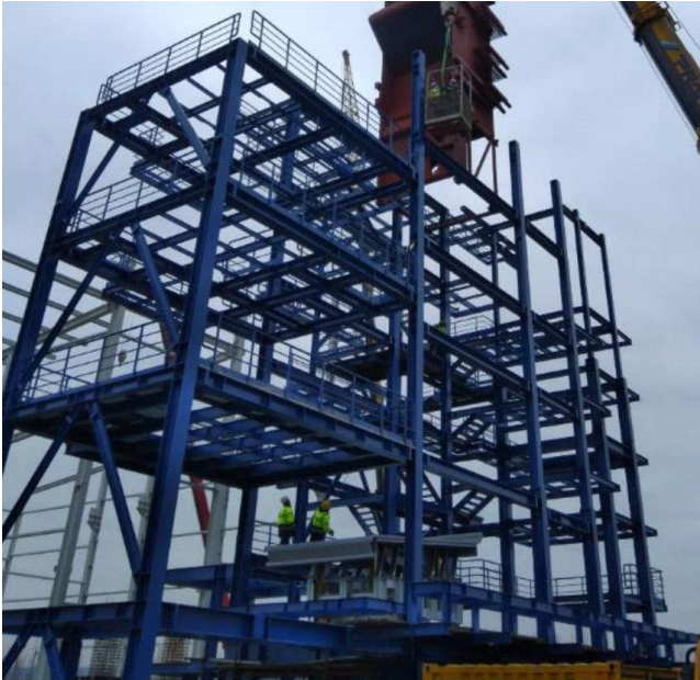
Fig. 2 Supporting steel structure
