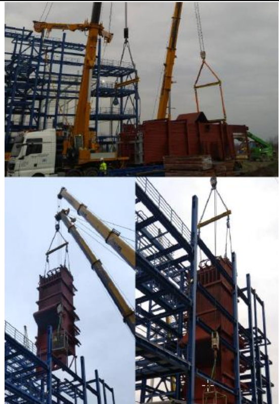
Fig. 4 Attaching the boiler module to cranes, its lifting, rotation and placement in the load-bearing steel structure.
