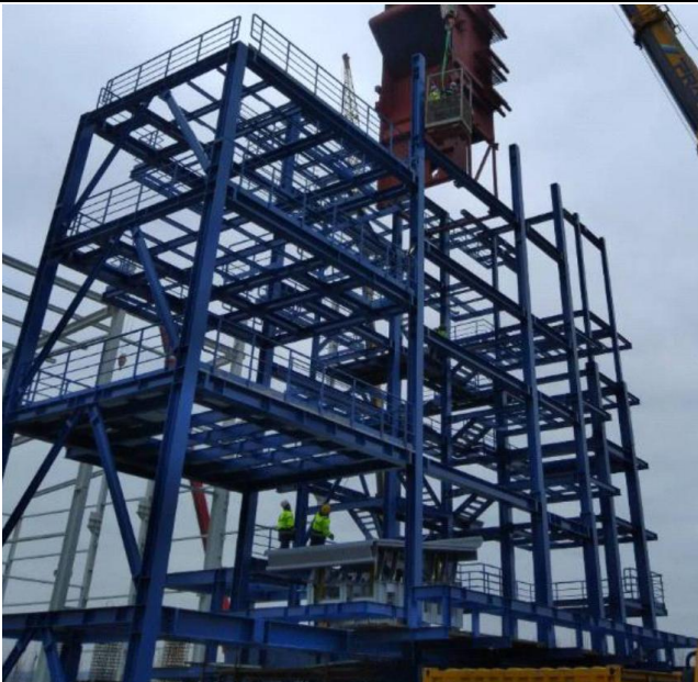
Fig. 2 Supporting steel structure
