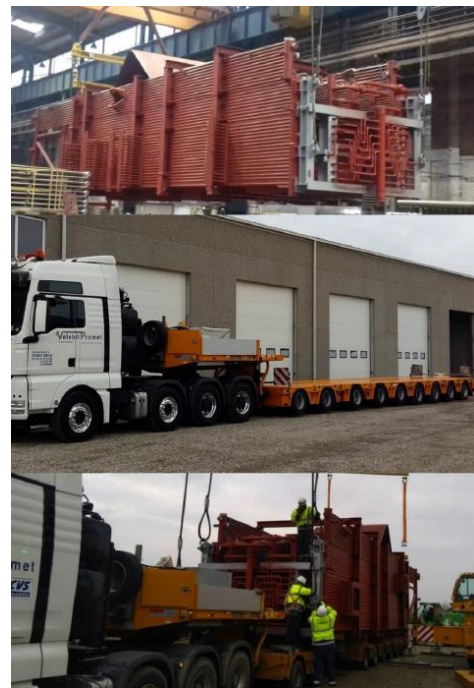
Fig. 1 Steam boiler module transport
