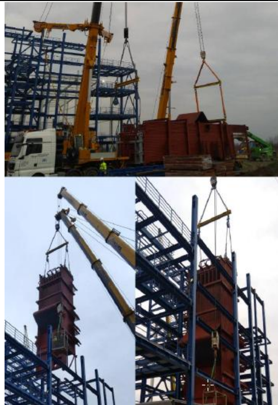
Fig. 4 Attaching the boiler module to cranes, its lifting, rotation and placement in the load-bearing steel structure.
