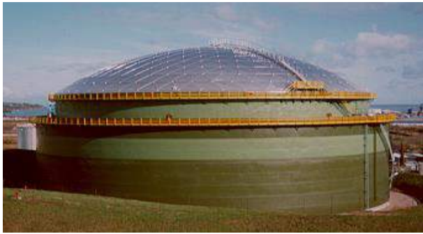
Figure 1. Reservoir for liquid natural gas manufactured from steel Niomol 490K.
