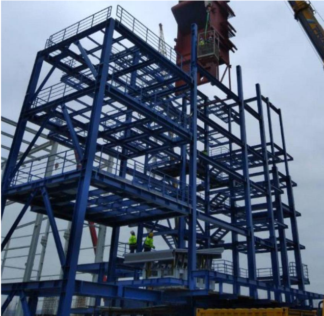
Fig. 2 Supporting steel structure
