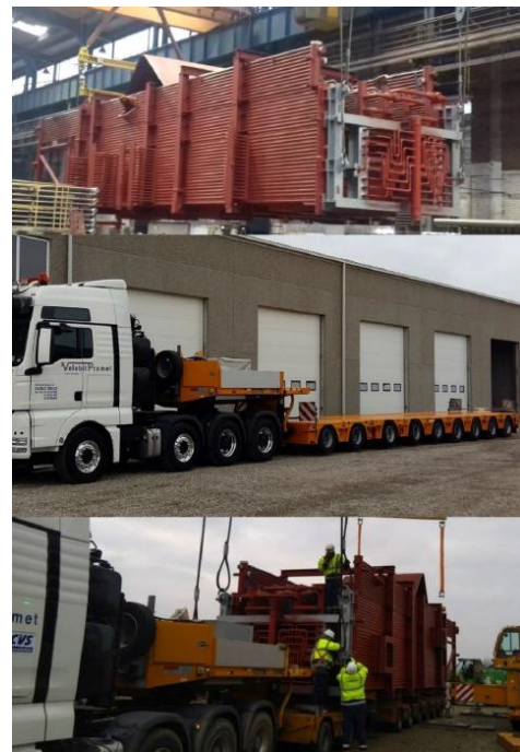
Fig. 1 Steam boiler module transport
