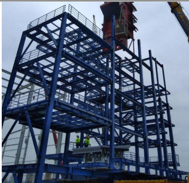
Fig. 2 Supporting steel structure
